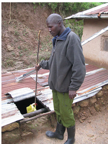
Aryatuha Bashil, a community-based trainer from Kagunga Parish in Uganda, demonstrates a do-it-yourself rain catchment cistern.
