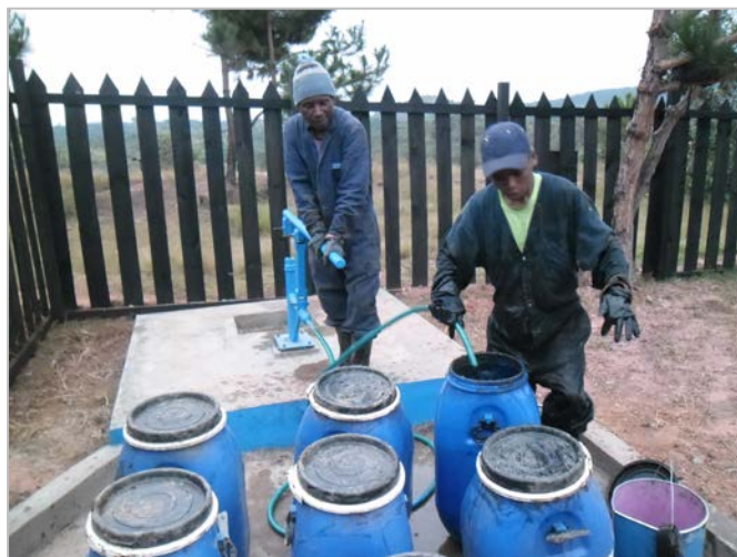
Workers from the local service provider, Aina, disinfect equipment used to extract and transport sludge to a burial site. The availability of water at the burial site is critical to ensure hygienic conditions.
